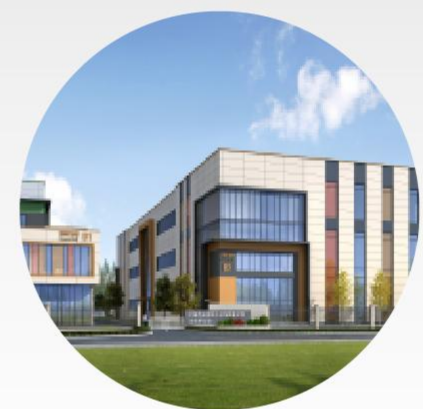
Hangzhou Bay Standard Factory
