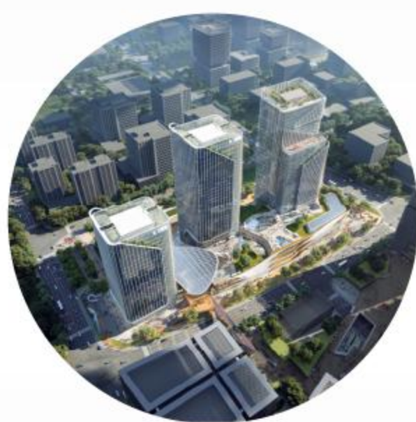
Zhangjiang Electricity Harbor
